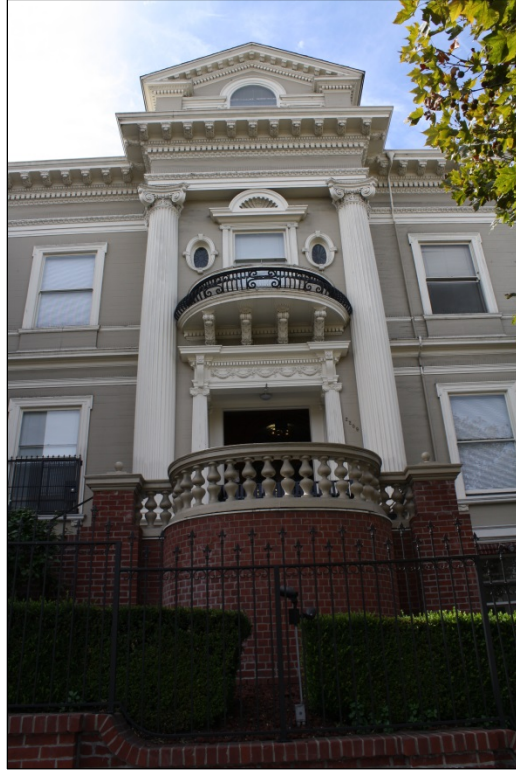
Figure 334. 2209 Van Ness Avenue, close up of the Classical Revival details on the primary elevation.
