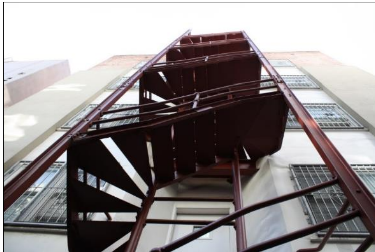
Figure 19. 1080 Bush Street, southern perspective of the north elevation. (Source: SWCA)
