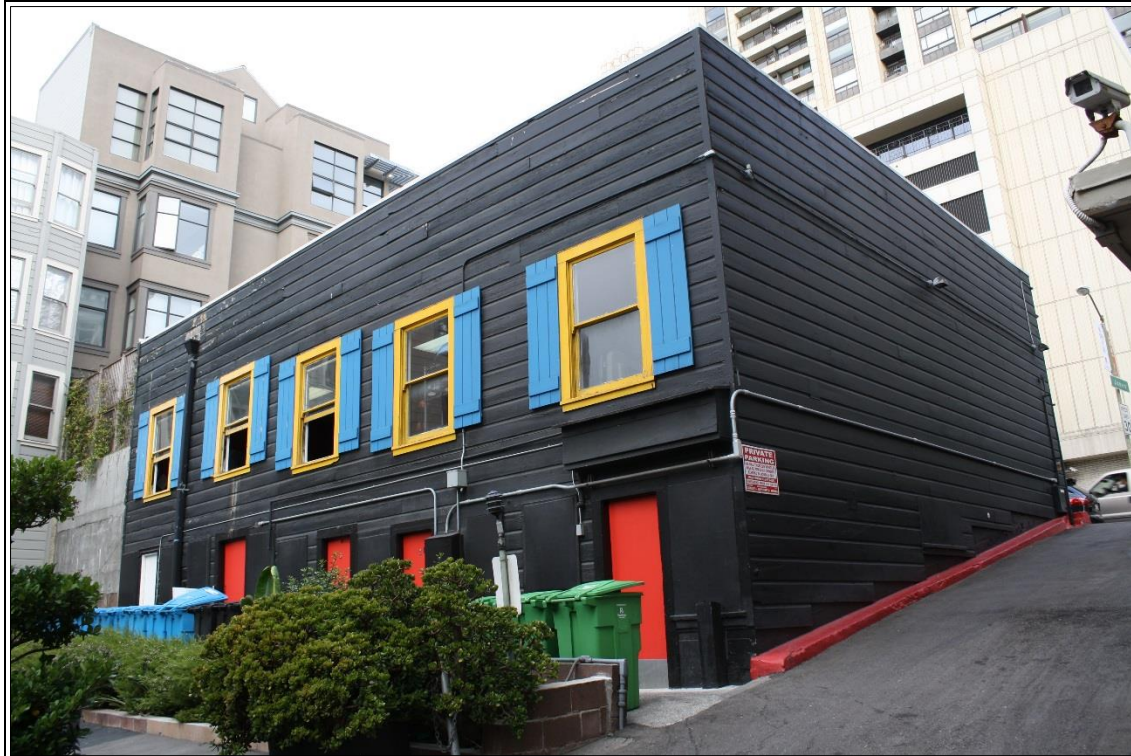
Figure 6. South and east facades, 1069 Pine Street. Source: SWCA, 2015.
