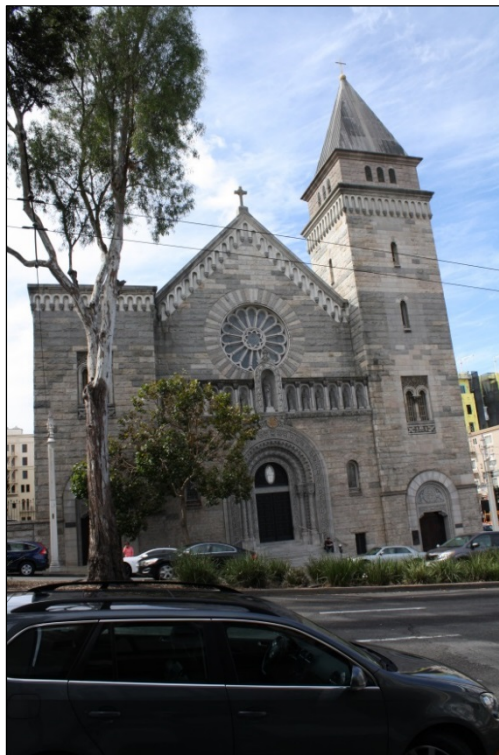
Figure 305. 2151 Van Ness Avenue, primary elevation.
