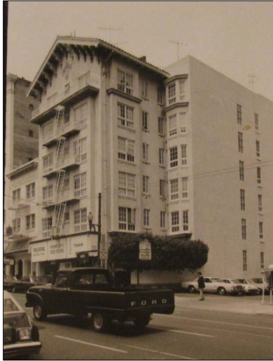
Figure 200. 1978 photo of 680 Sutter Street. (Source: San Francisco Heritage)
