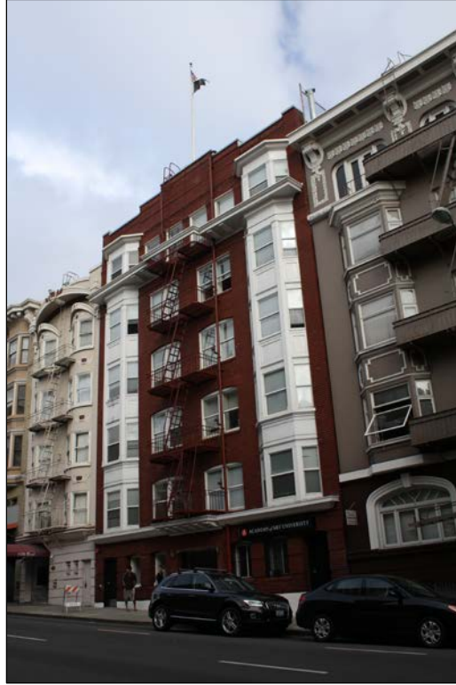
Figure 14. 1080 Bush Street, detail. (Source: SWCA)
