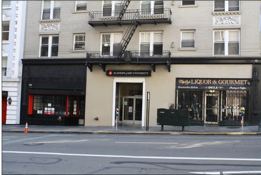
Figure 175. 655 Sutter Street, first story of the primary elevation.
