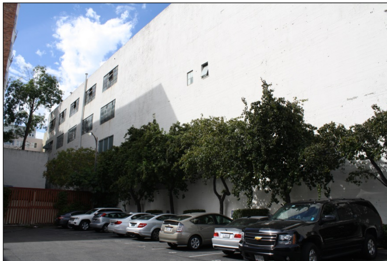
Figure 289. 1849 Van Ness Avenue, northwestern perspective of the southern elevation.
