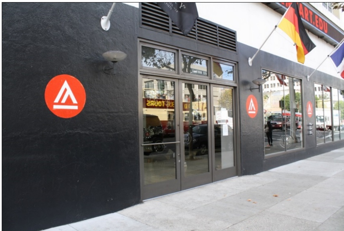
Figure 283. 1849 Van Ness Avenue, close up of the main entry on the primary elevation.
