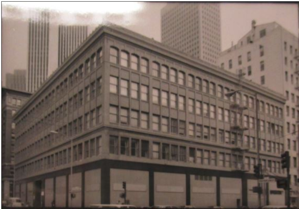
Figure 66. 1977 photograph of 77-79 New Montgomery Street. (Source: San Francisco Architectural Heritage Survey)
