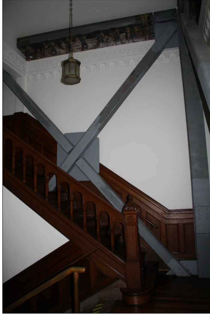
Figure 316. Interior seismic bracing installed in stairwells and hallways off the main nave of subject property.
