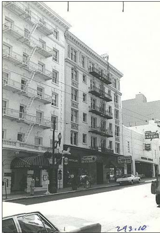
Figure 181. 1976 photo of 655 Sutter Street. (Source: San Francisco Heritage)
