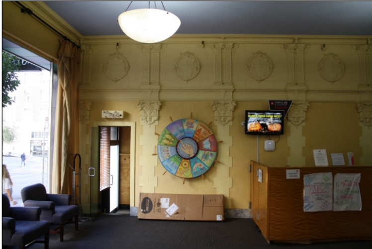
Figure 214. Interior lobby of subject property.
