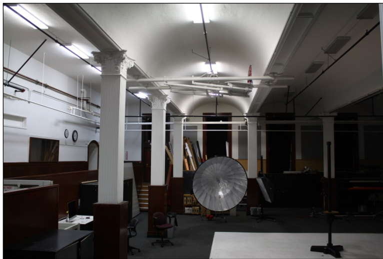
Figure 317. Interior basement of subject property.
