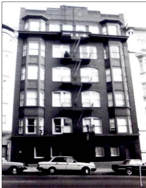
Figure 26. 1989 photo of 1080 Bush Street. (Source: SF Planning Department, Anne Bloomfield 1989 Survey.)
