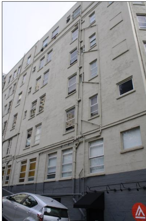
Figure 95. 1055 Pine Street, northeast perspective, west elevation. (Source: SWCA)
