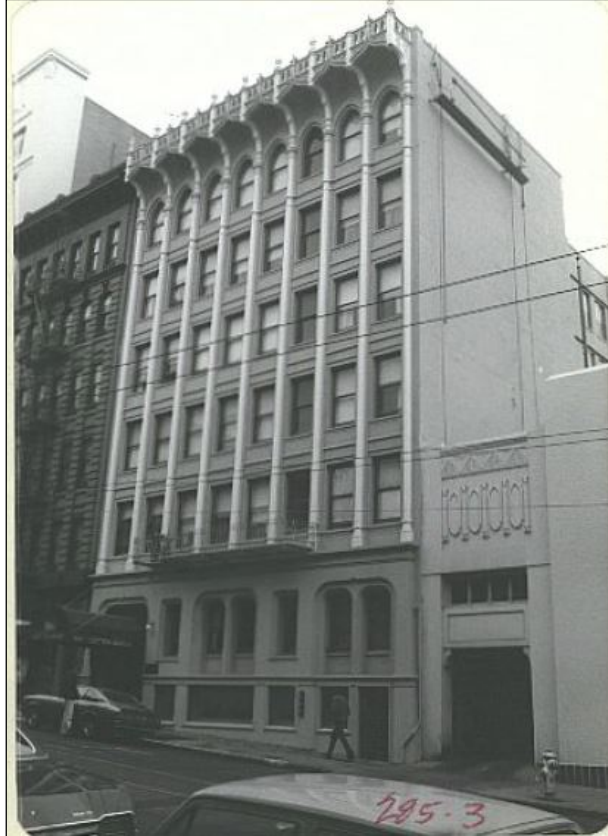
Figure 237. 1976 photo of 860 Sutter Street. (Source: San Francisco Heritage)
