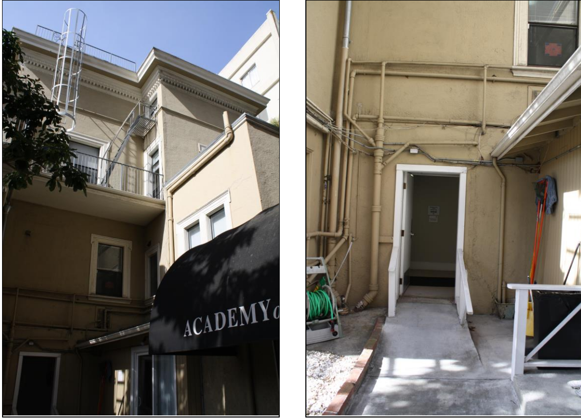
Figure 7. East façade, 1916 Octavia Street. Source: SWCA, 2015.
