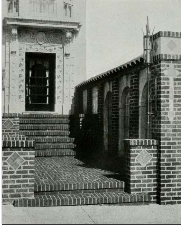
Figure 198. 1919 photo of 680 Sutter Street. (Source: Architect and Engineer , September 1919)
