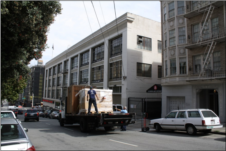
Figure 287. 1849 Van Ness Avenue, southeastern perspective of the north and west elevations.
