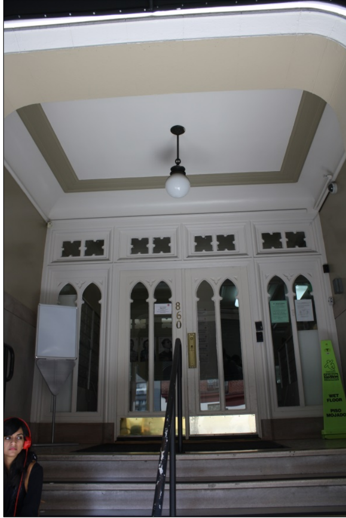
Figure 228. 860 Sutter Street, close up of the main entry on the primary elevation.
