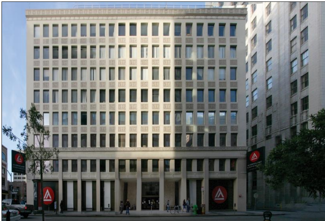
Figure 84. 1995 photograph of 180 New Montgomery Street. (Source: AAU, 1995)
