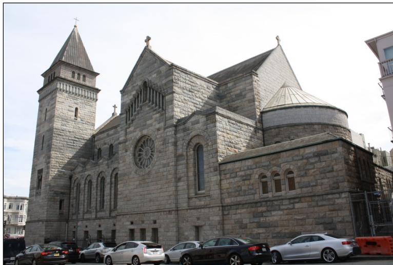
Figure 309. 2151 Van Ness Avenue, southeastern perspective of the north and west elevations.
