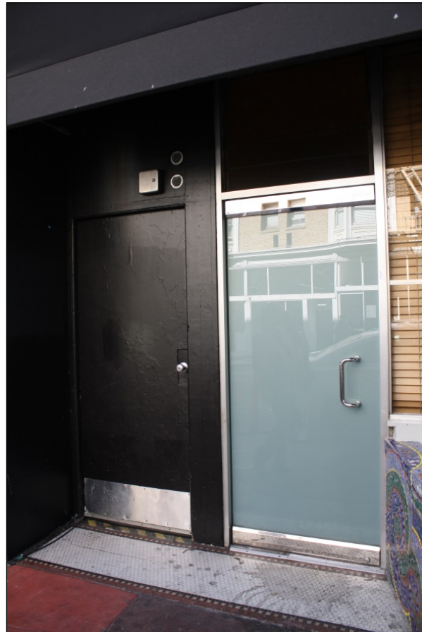
Figure 210. 817-831 Sutter Street, close up of the entry to the former café and basement on the primary elevation.
