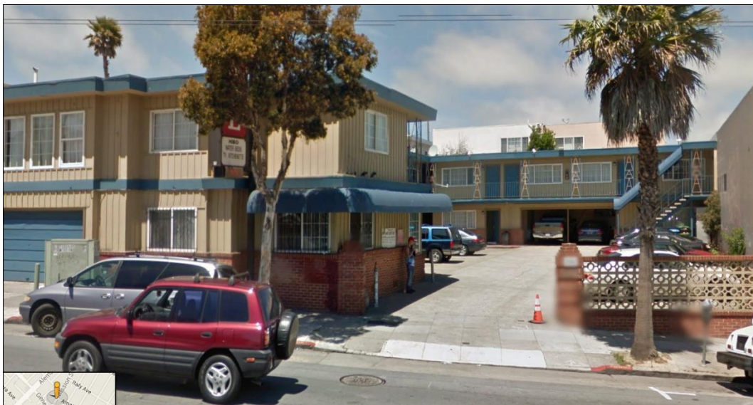
Figure 51. Amazon Motel, 2015. Source: Google.
