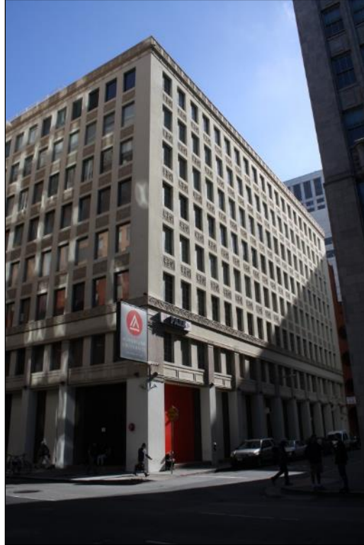
Figure 78. 180 New Montgomery Street, southeast perspective of the northwestern elevation. (Source: SWCA)
