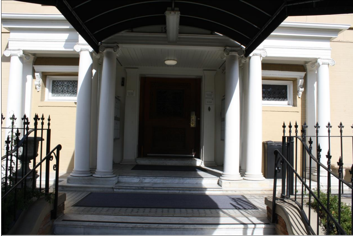
Figure 5. South façade, primary entrance, 1916 Octavia Street. Source: SWCA, 2015.
