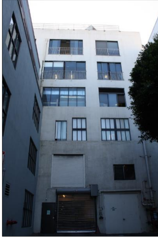
Figure 50. 58-60 Federal Street, southwestern perspective of the northeastern elevation. (Source: SWCA)
