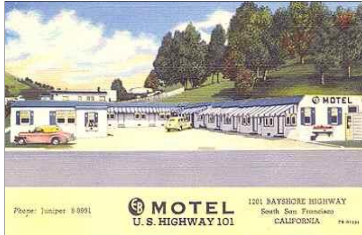
Figure 19. E.B. Motel, 1201 Bayshore Highway, San Francisco (not extant). Source: 101Cafe.net.
