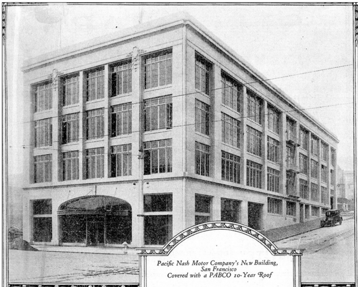
Figure 293. 1921 photo of 1849 Van Ness Avenue. (Source: Architect and Engineer , January 1921)
