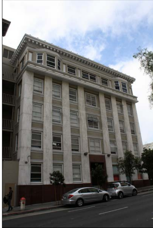
Figure 91. 1055 Pine Street. (Source: SWCA)
