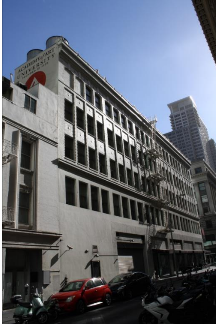
Figure 61. 77-79 New Montgomery Street, secondary elevation along Jesse Street. (Source: SWCA)
