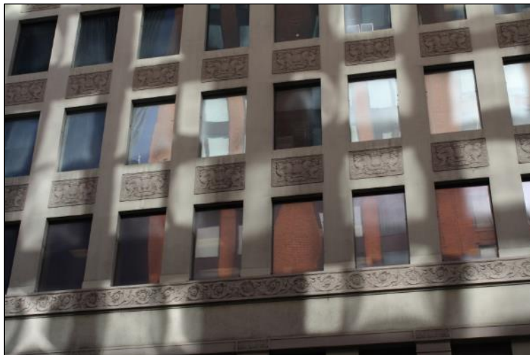
Figure 76. 180 New Montgomery Street, detail, windows and terra cotta spandrel panels. (Source: SWCA)
