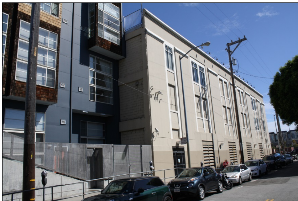
Figure 274. 466 Townsend Street, southeastern perspective of the southwestern and northwestern elevations.
