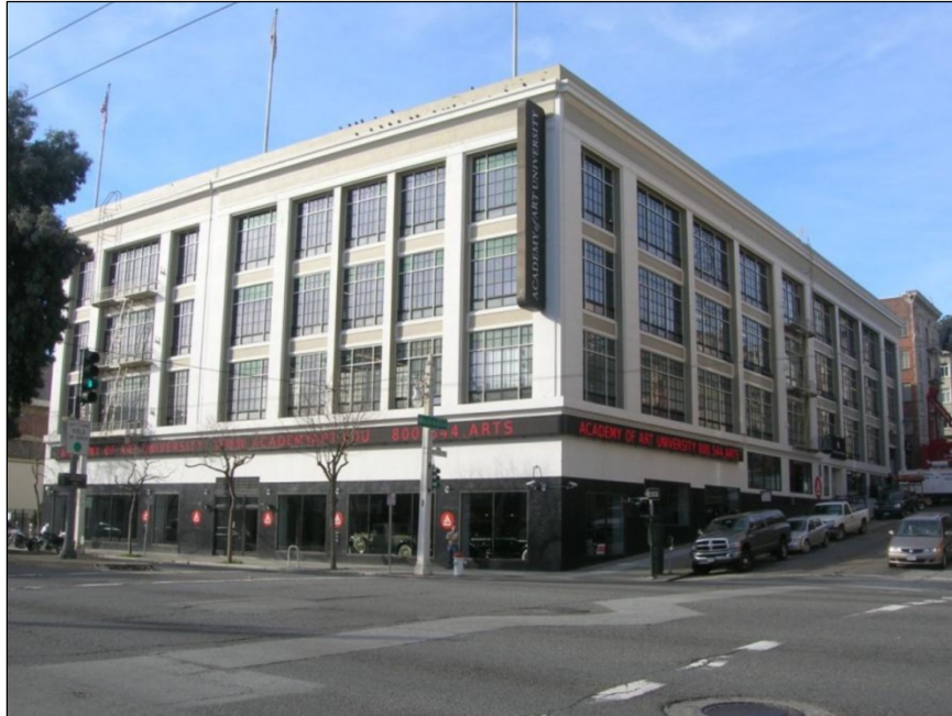
Figure 296. 2011 photo of 1849 Van Ness Avenue. (Source: Atkins)
