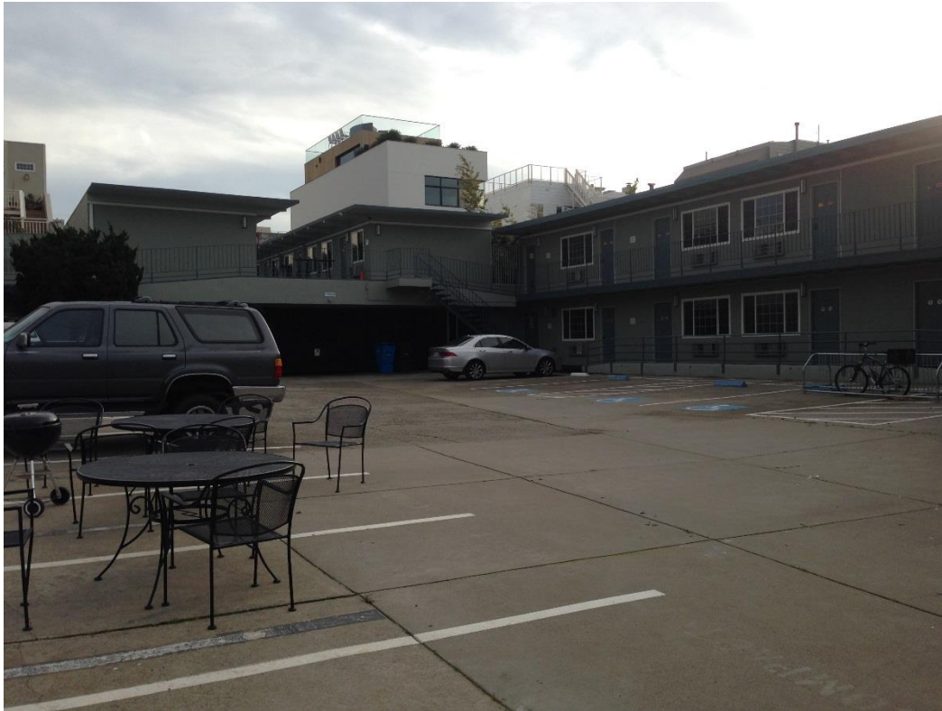
Figure 5. West and south wings (1960) Star Motel, 1727 Lombard Street, 2015 (Source: SWCA).
