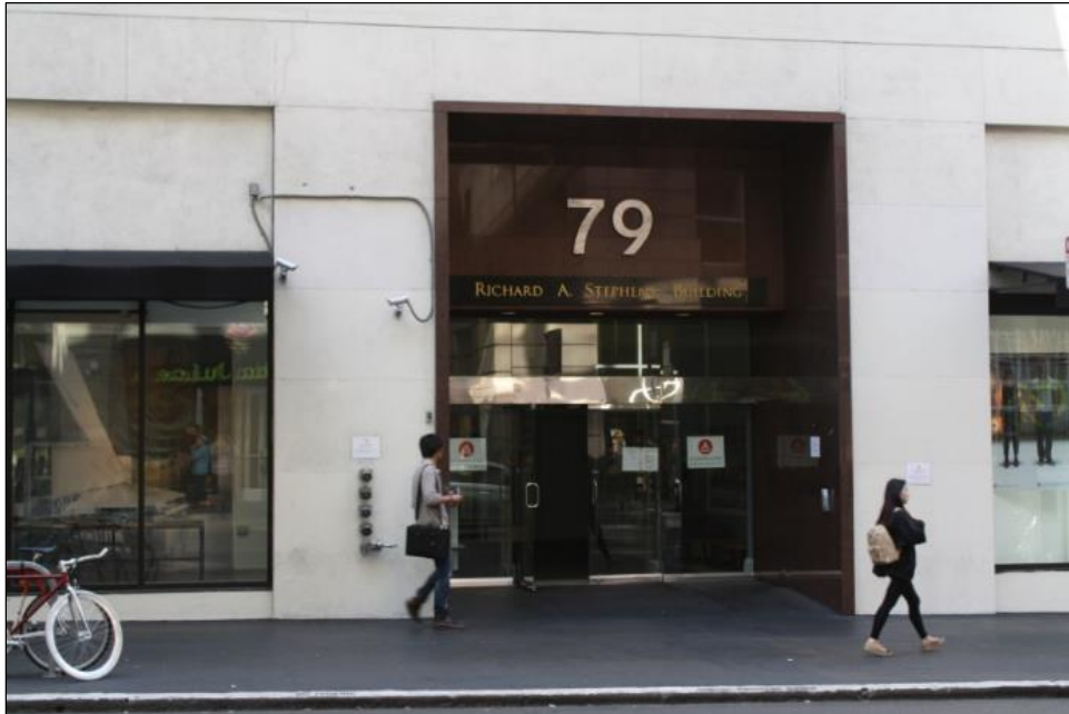
Figure 60. 77-79 New Montgomery Street, detail, principal entrance. This entrance represents a 1960 remodel carried out by renowned San Francisco architect Gardner A. Dailey for Allied Properties. (Source: SWCA)
