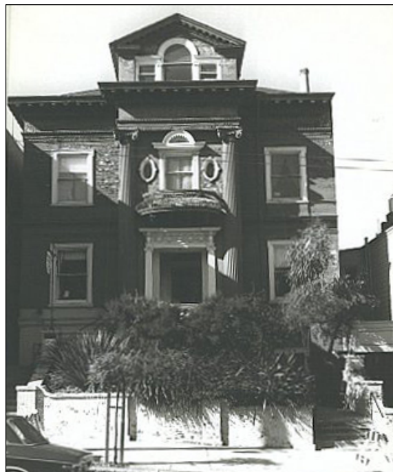
Figure 342. 1976 photo of 2209 Van Ness Avenue. (Source: San Francisco Planning Department)
