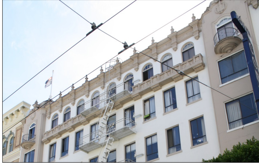
Figure 211. 817-831 Sutter Street, close up of the upper story details.
