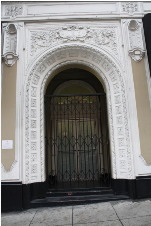
Figure 165. 625-629 Sutter Street, close up of the main entry on the primary elevation.
