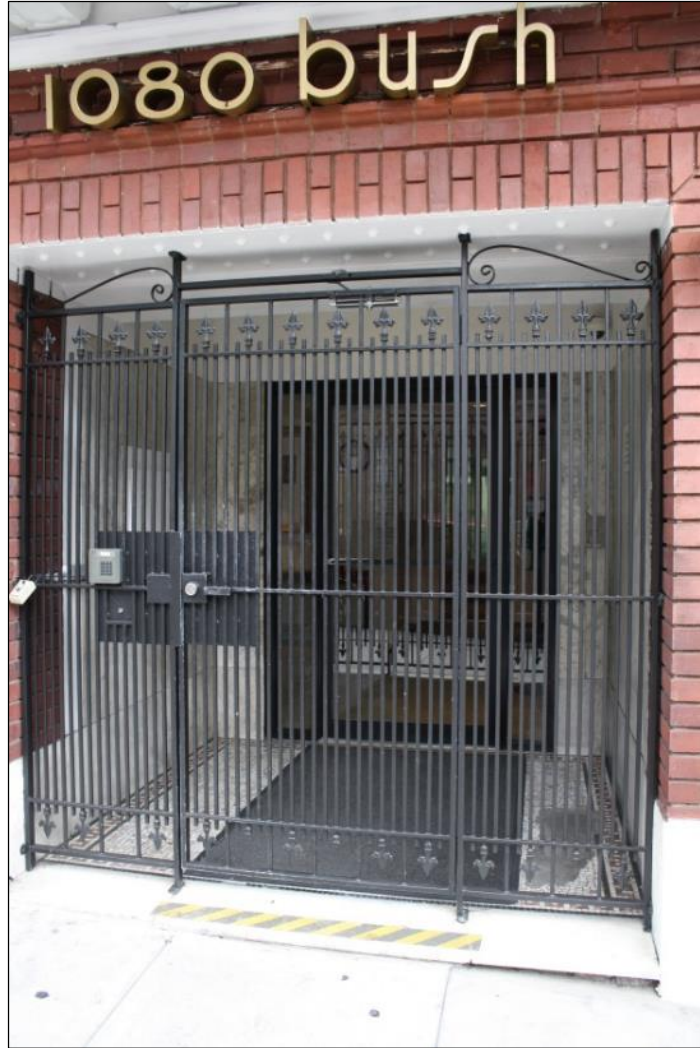
Figure 17. 1080 Bush Street, detail, main entry on the primary elevation. (Source: SWCA)
